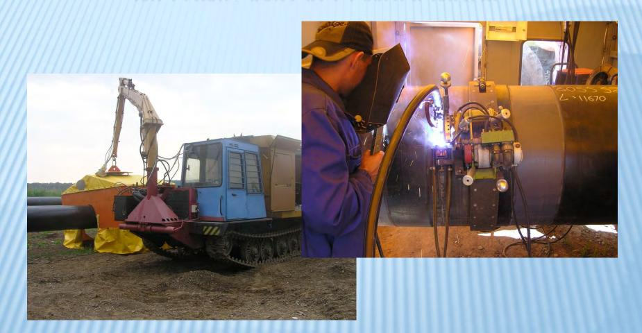
Welding gas pipeline Automatic welding flux cored wire
