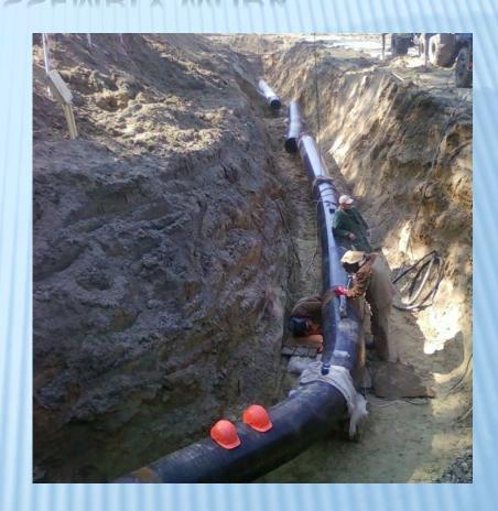
Welding pipeline Electric Arc welding method
