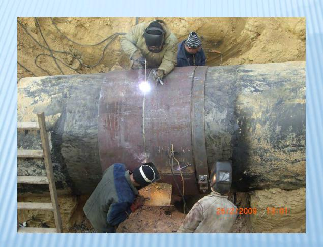
Gain the carrying capacity of welded coupling
