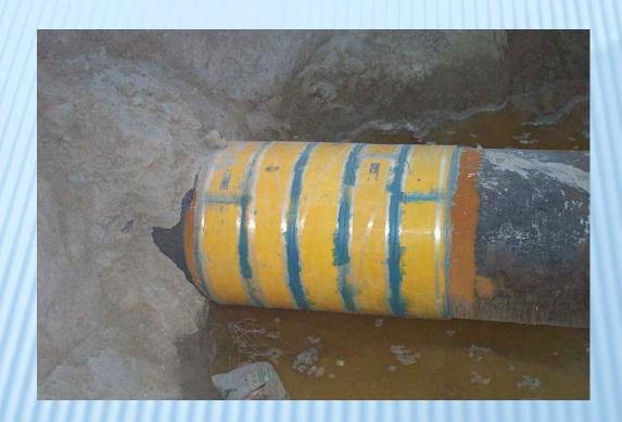
Bearing capacity of composite gain bandage
