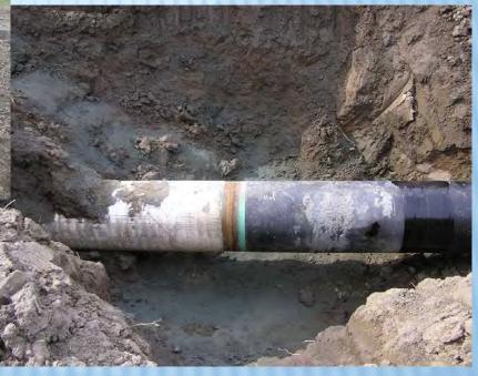
Construction crossing under the river, DN 700, 650m Horizontal Directional Drilling method
