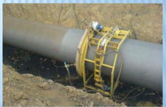
Equipment to remove old coatings surface preparation and application of new insulation coating
