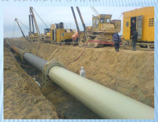
Applying polyurethane insulation coating Complex repair of pipelines
